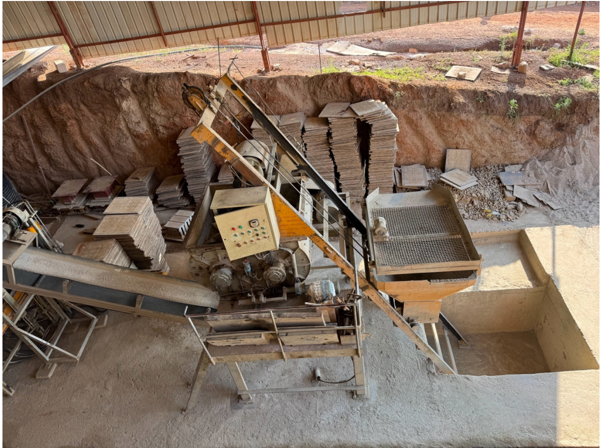
Figure 11. On-site maker yard for blockwork (2025). © Julia Backhaus.
