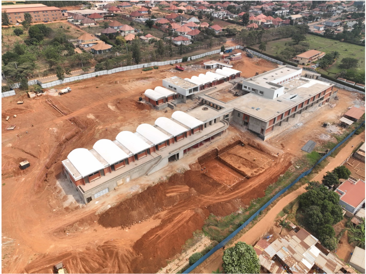
Figure 6. Drone image of the construction site above the valley, July 2026. © Julia Backhaus.
