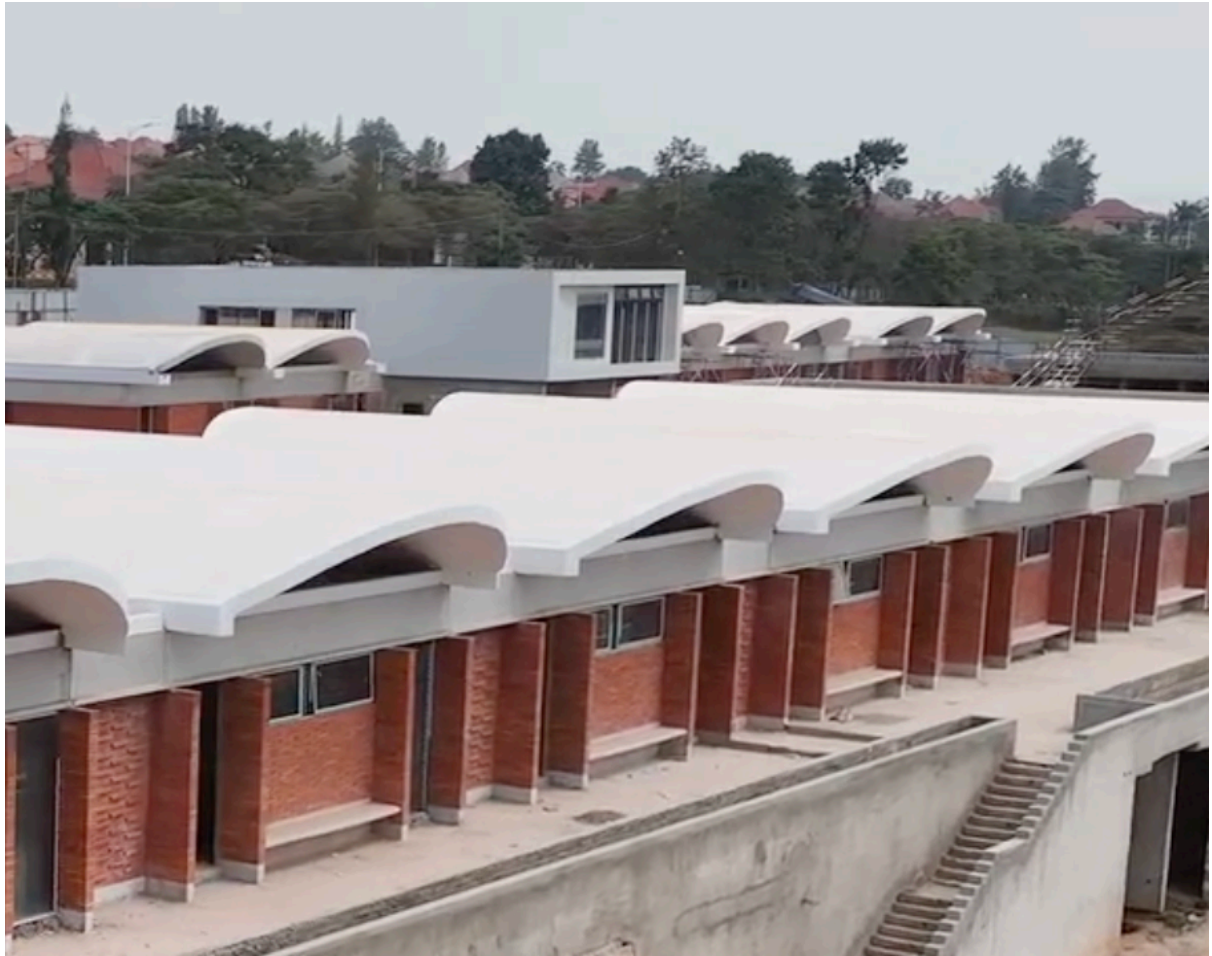
Figure 9. Double-skin vaulted roof structure over the inpatient ward. Photograph, 2026. © Julia Backhaus.
