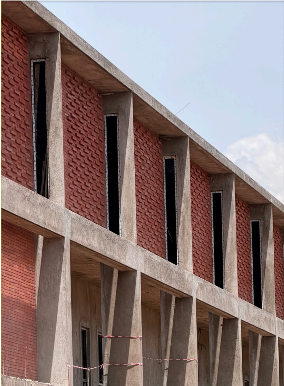
Figure 12. Brick façade detail under construction (2026). © Julia Backhaus.
