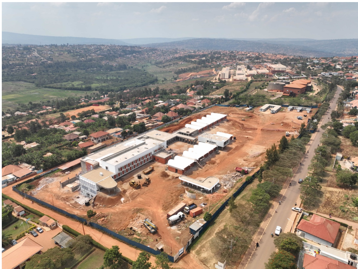
Figure 13. Drone image of the Centre under construction July 2026. © Julia Backhaus.
